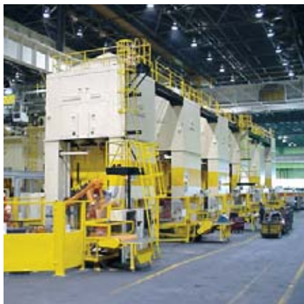
Permanently fixed gantries, ladders and walkways are incorporated into this machinery and equipment to reduce the risk of a fall from height occurring during operation and maintenance.
